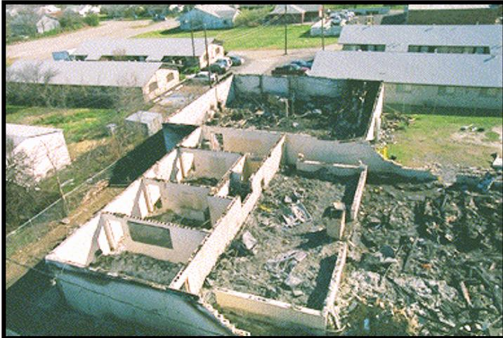
A fire in a single-story church building resulted in the deaths of three fire fighters after a collapse of the truss roof system.
